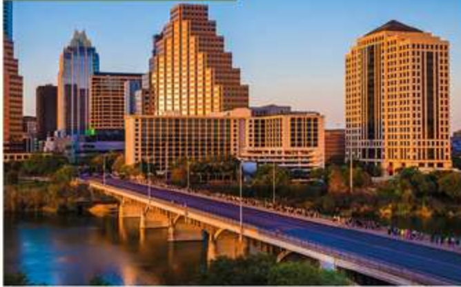
Congress Avenue Bridge Austin, Texas
